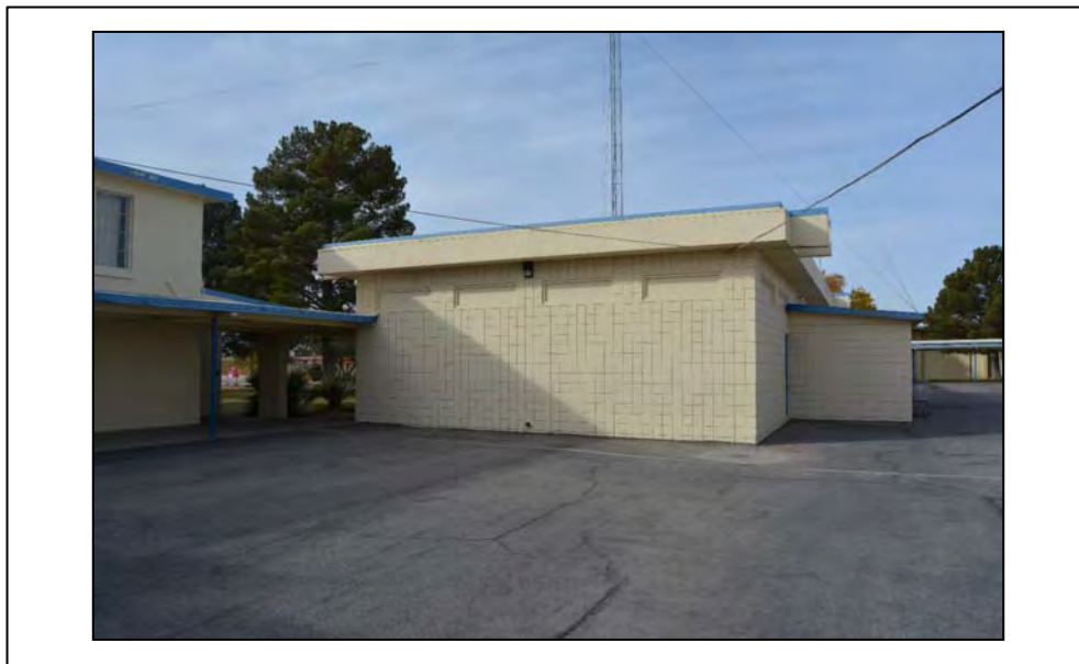
Façade: East Facing: W Photographer: Serra Akboy-İlk Date: 12/11/16
