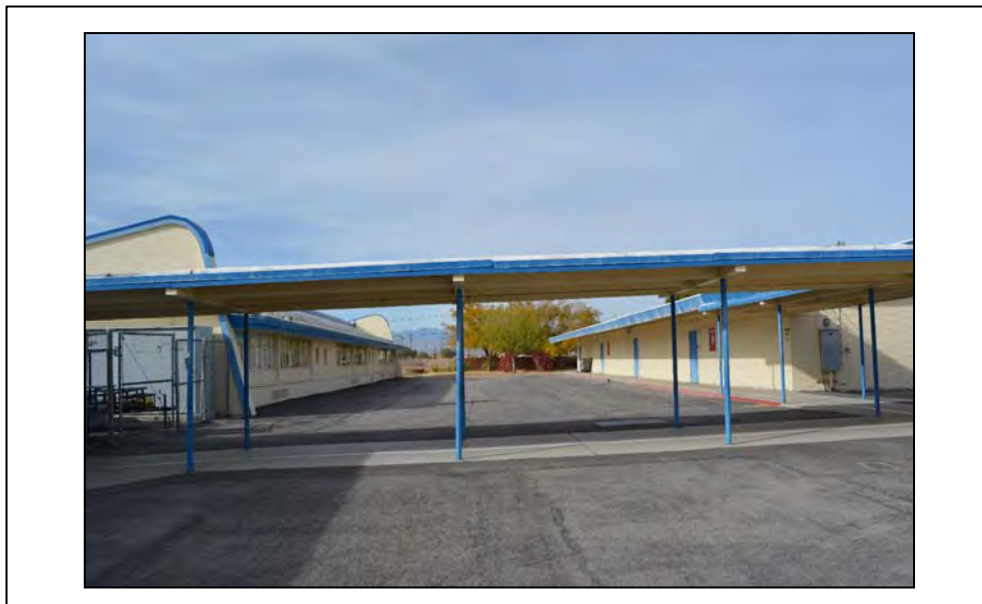
Façade: North (left bldg) Facing: W Photographer: Serra Akboy-İlk Date: 12/11/16
