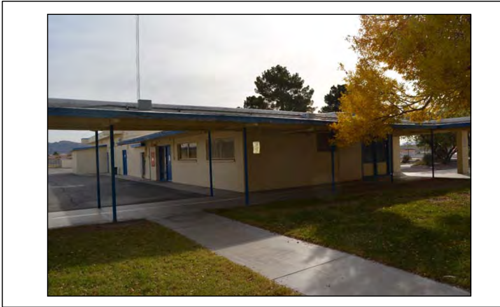
Façade: West and North Facing: SE Photographer: Serra Akboy-İlk Date: 12/11/16
