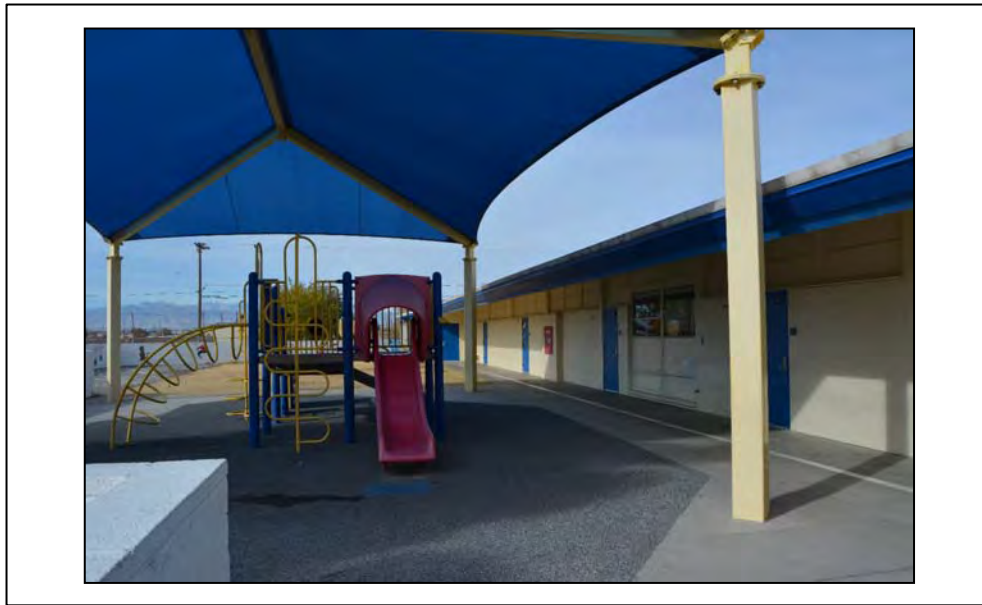
Façade: South Facing: W Photographer: Serra Akboy-İlk Date: 12/11/16
