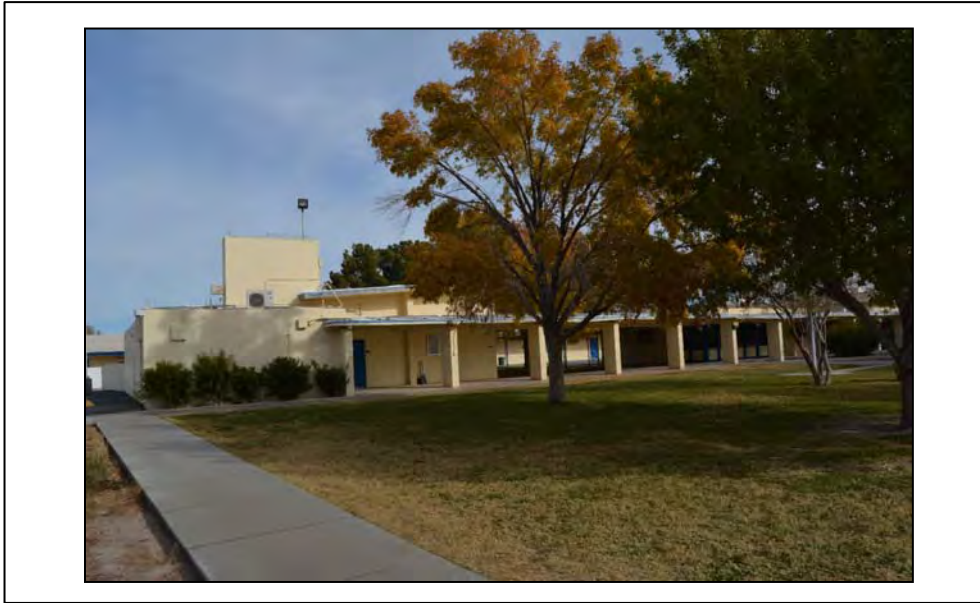
Façade: N/A Facing: N Photographer: Serra Akboy-İlk Date: 12/11/16
