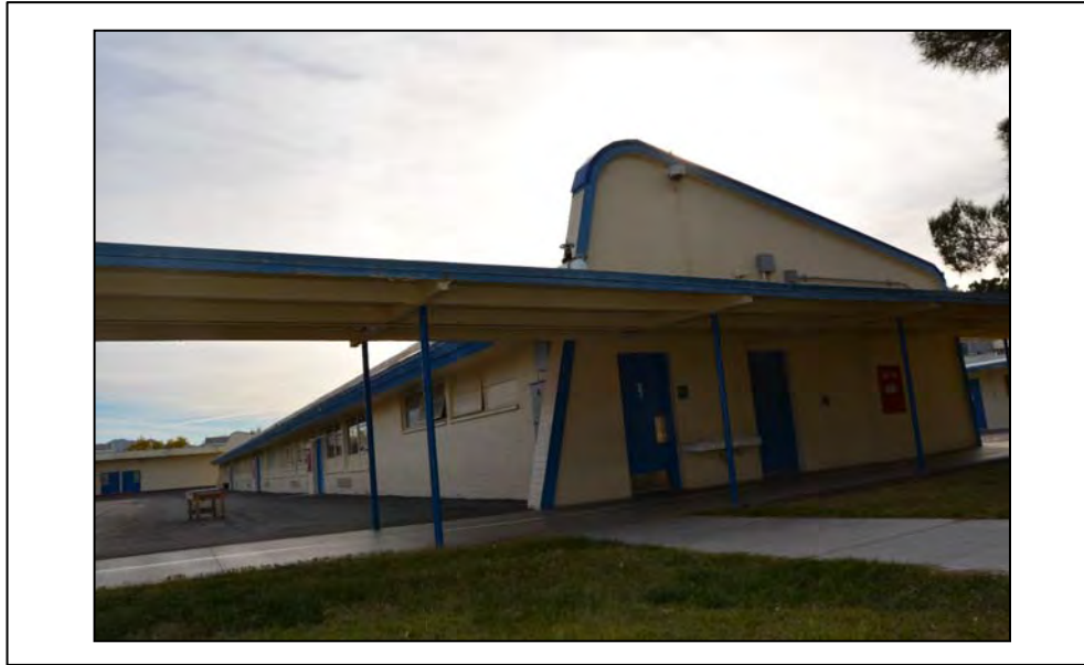
Façade: West Facing: N Photographer: Serra Akboy-İlk Date: 12/11/16
