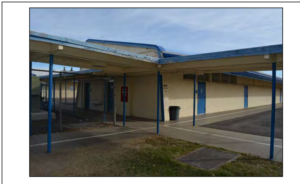
Façade: West and South Facing: NE Photographer: Serra Akboy-Ilk Date: 12/11/16
