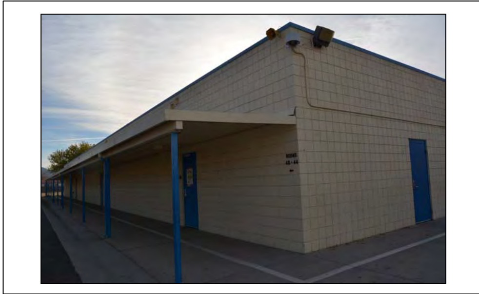
Façade: North Facing: SE Photographer: Serra Akboy-Ilk Date: 12/11/16
