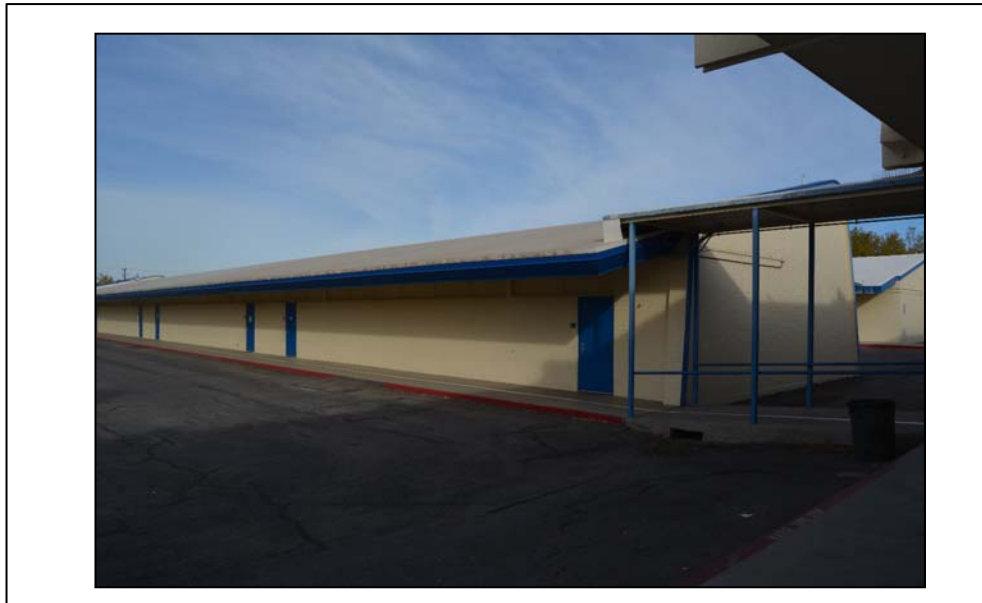
Façade: East and South Facing: NW Photographer: Serra Akboy-İlk Date: 12/11/16
